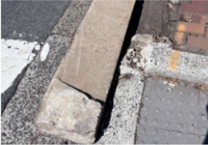
25) NW Coner of Franklin St & S Washington St Intersection(Req#279138)
